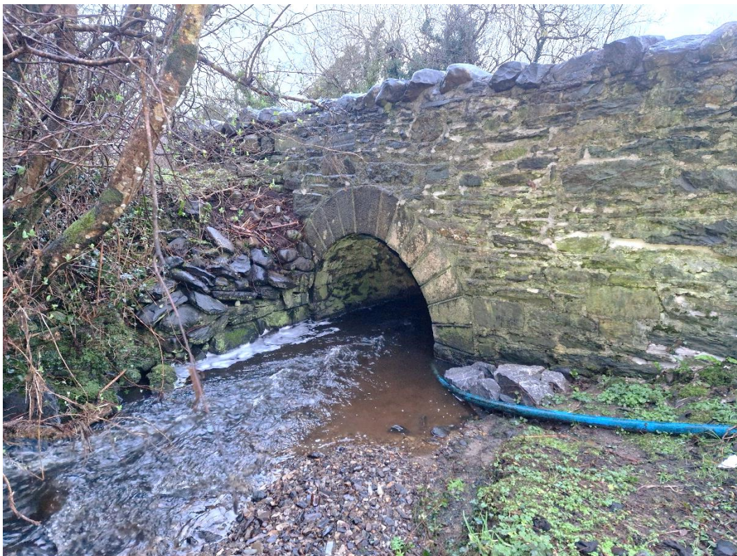
Figure 2-4 – Existing bridge south elevation
