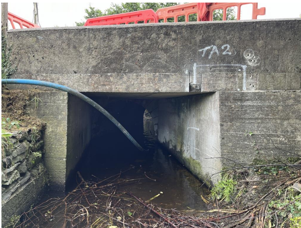
Figure 2-5 – Existing bridge north elevation
