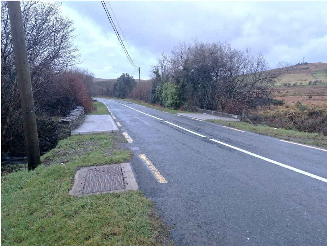
Figure 2-3 – Existing bridge surface looking west
